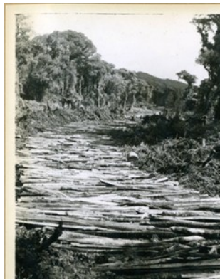
Photo of corduroy road construction, Puerto Rico mtns 1940-41
